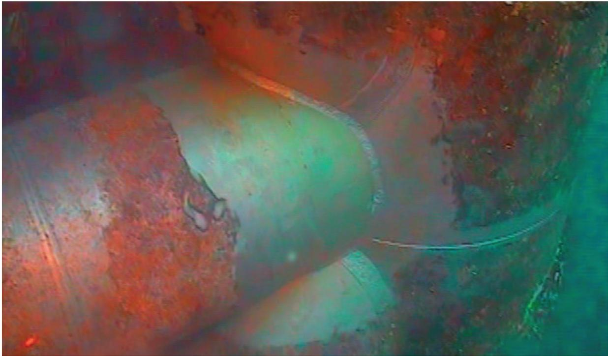
**FIG 3: Horizontal Member to Jacket Leg forming a KT Connection on a typical offshore structure.**
