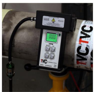
Additionally, a remote flow control box can be connected to the output of the HPM, which allows for automated purging of any inert welding gas. Control of purge gas flow ensures quick, accurate, and efficient purging, which can improve the quality of welds, reduce the risk of weld failures, and save money on purge gas.
